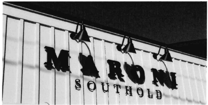
Above: Downward facing gooseneck lighting
